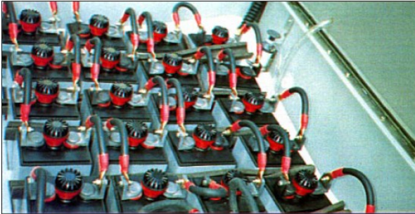
Fig.7 – Connections of batteries arrays
